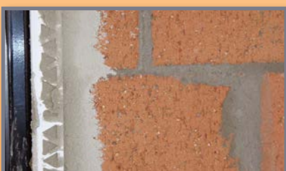
Patch render locks the angle on the corner
