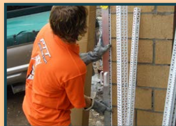
Suction will hold the trim in place & the levels will keep it straight
