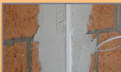
Expansion Joint rendered on the wall
